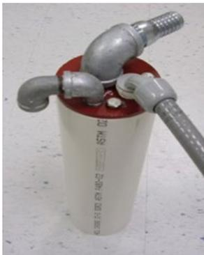
*NOTE: A one-piece top plate (shown in red in photo) must be used on a well that may be used on a well that terminates in an approved well house.*
